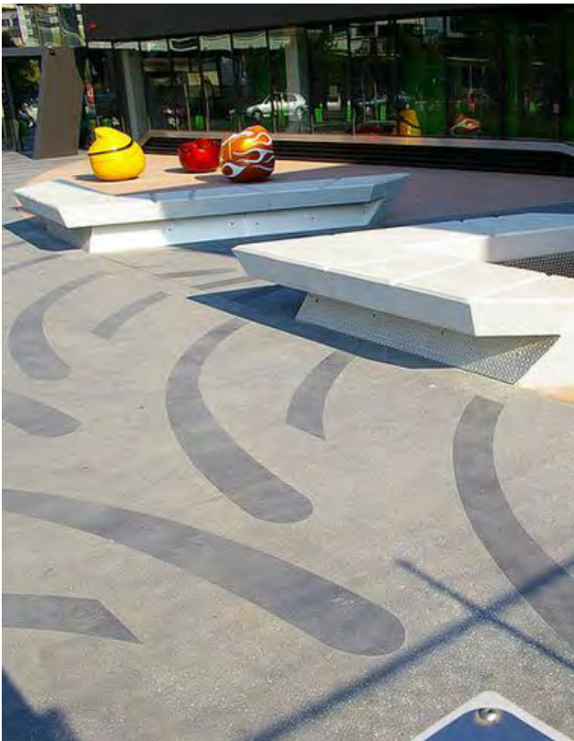
Sandblasting in concrete foot path
