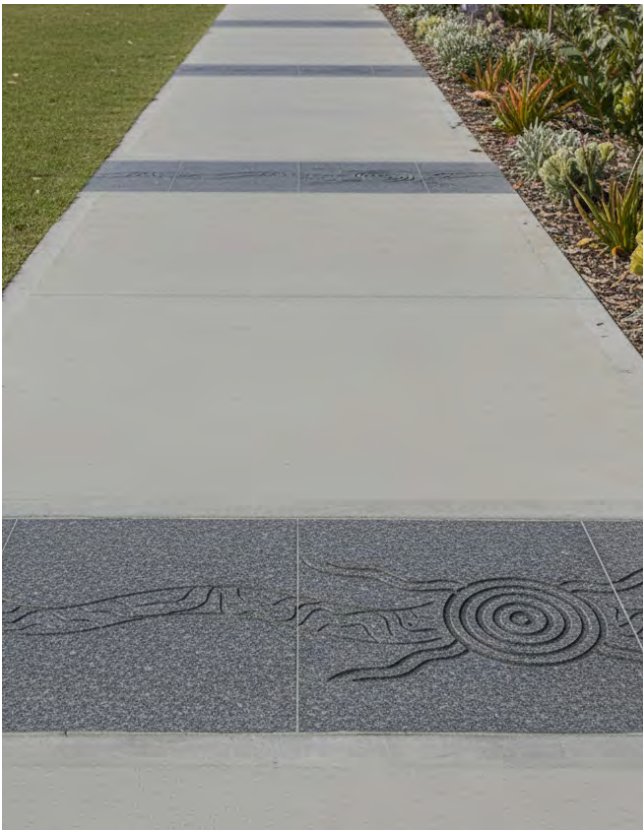
Paver inlays in concrete footpaths
