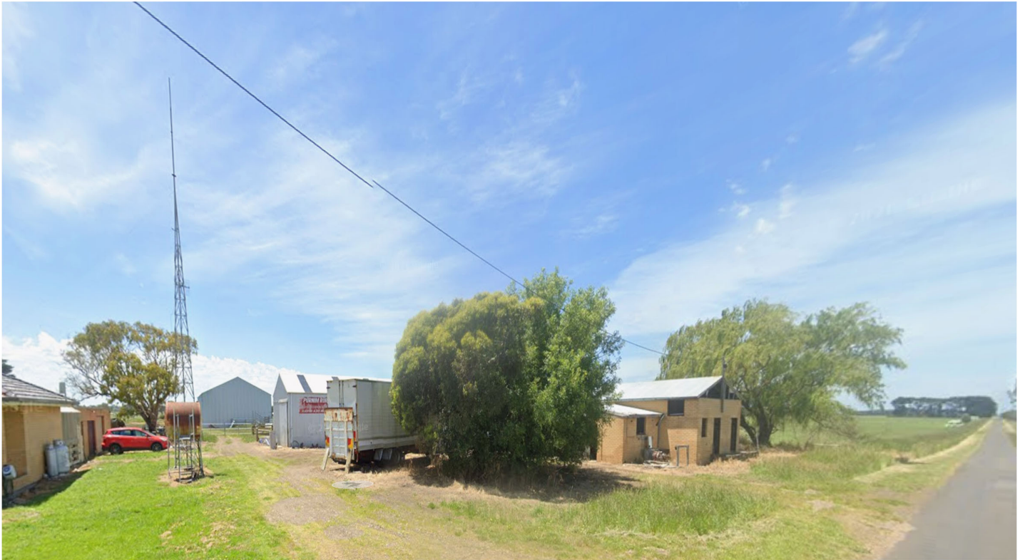
Redundant dairy and outbuildings with the excised dwelling
