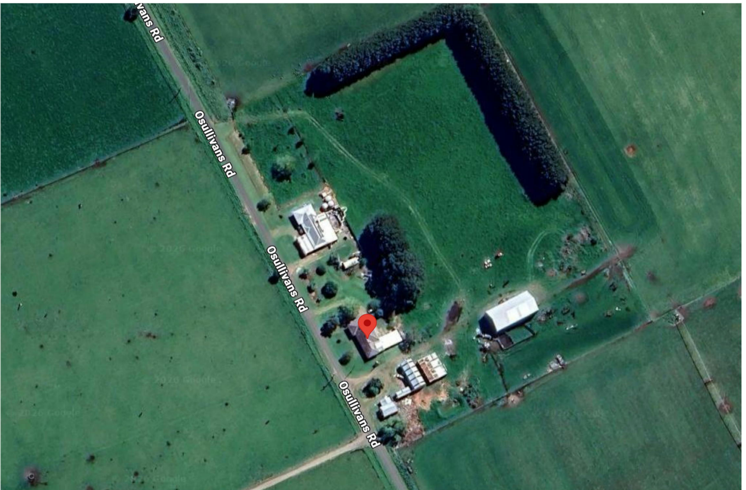
Subject dwelling aerial image
