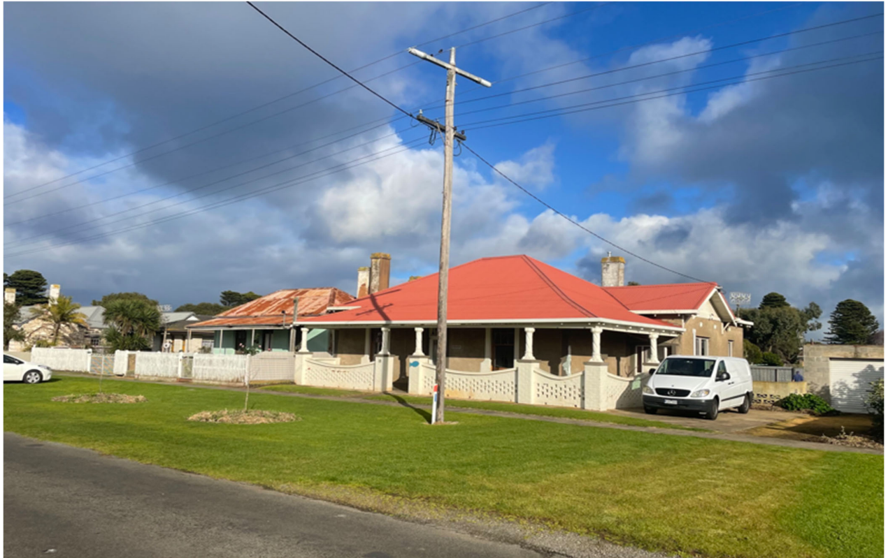
Subject dwelling frontage to James Street
