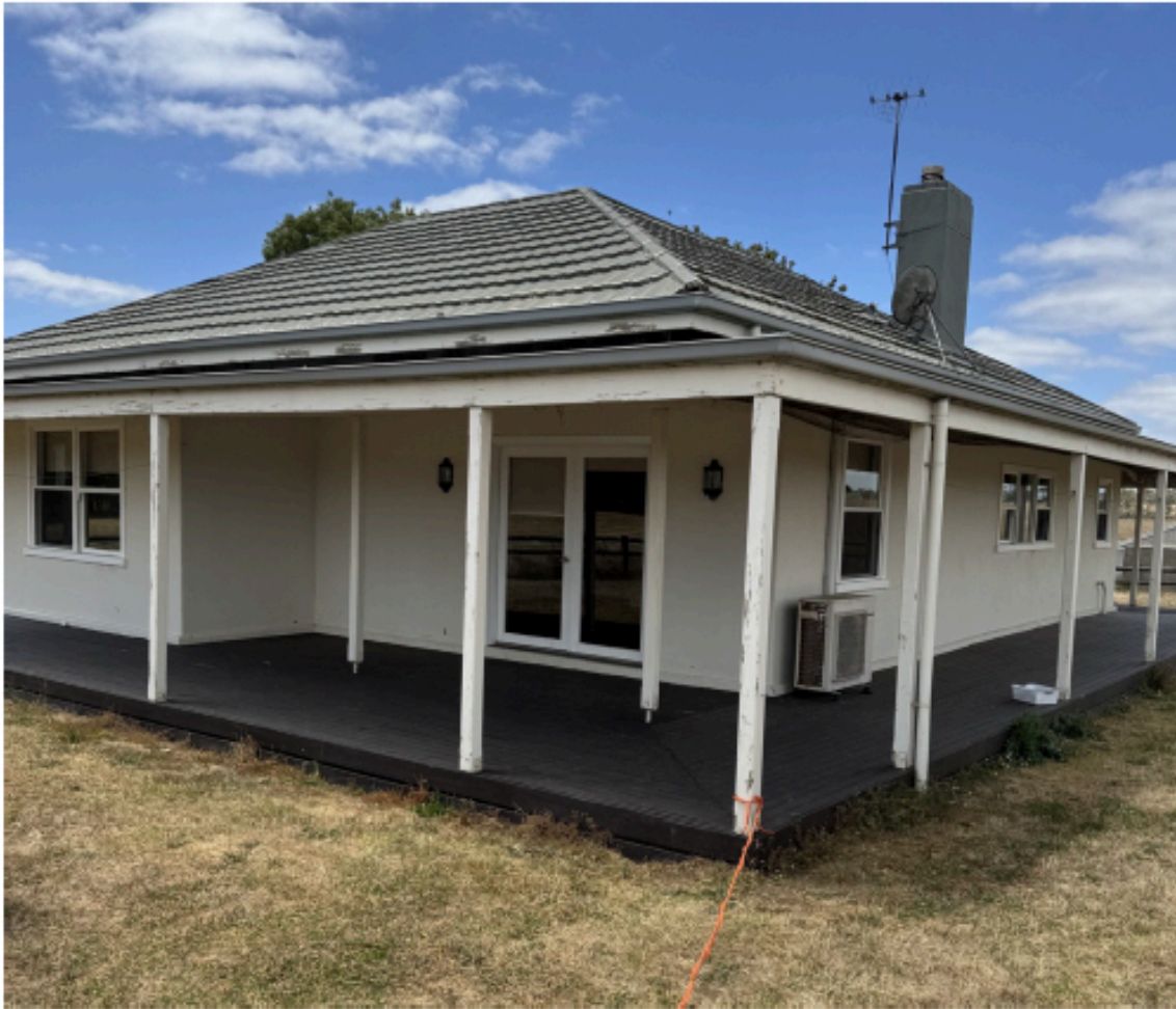
Image 5: View of existing house externally.
