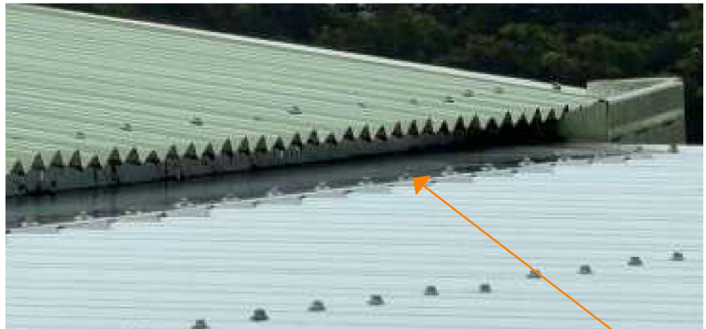
FLASHING BETWEEN CABIN ROOF & CARPORT ROOF EXISTING PHOTO
