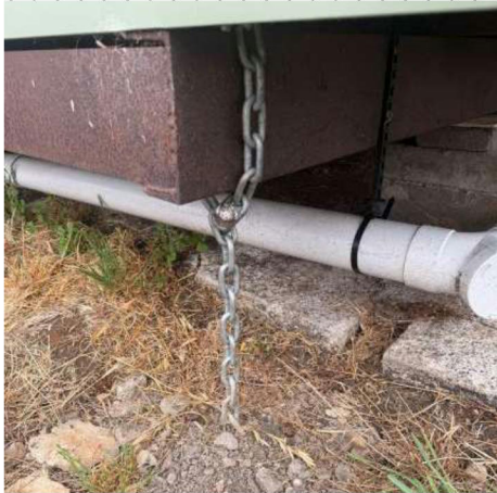
RING BEAM & CHAIN TIE DOWN EXISTING PHOTO
