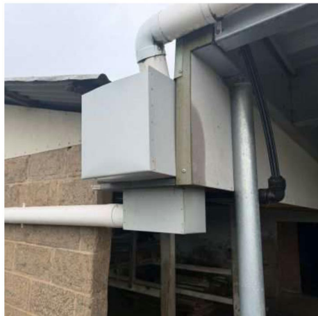
BOX GUTTER & SUMP EXISTING PHOTO
