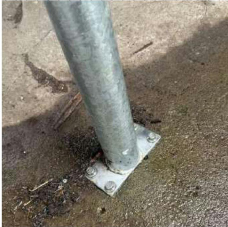
COLUMN TO SLAB CONNECTION EXISTING PHOTO
