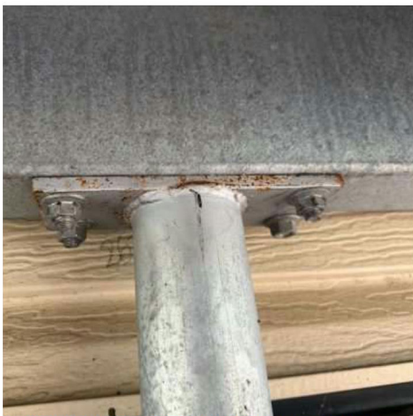
COLUMN TO BEAM CONNECTION EXISTING PHOTO
