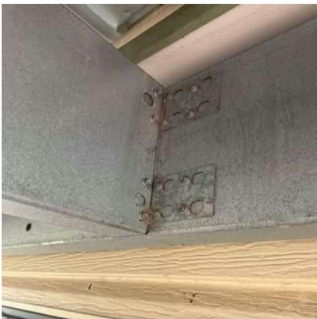
RAFTER TO BEAM CONNECTION EXISTING PHOTO
