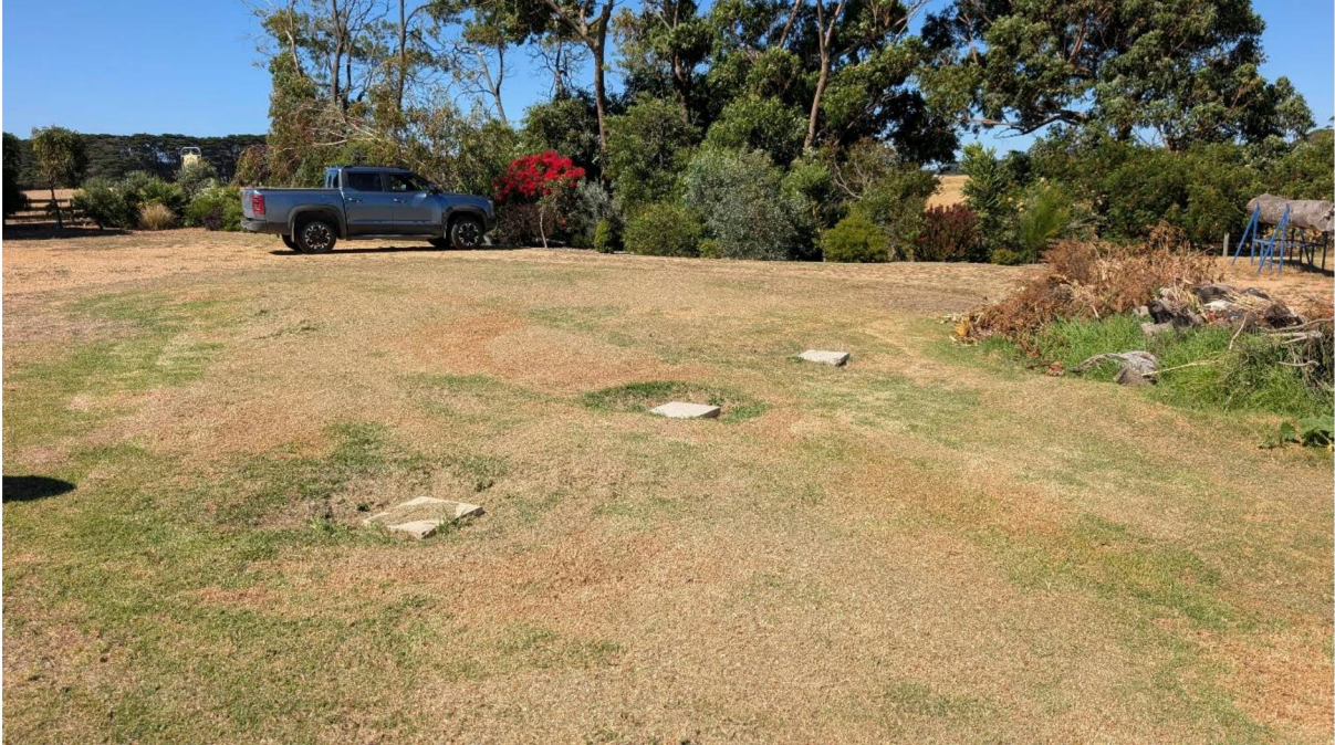
Image 11: Existing permitted effluent field.
