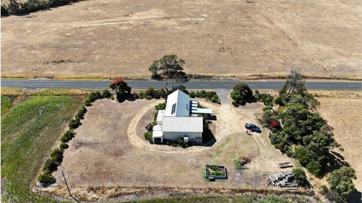
Images 7 & 8: Southern site and building aspect.
