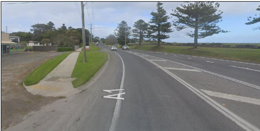
Figure 5: Princes Highway (facing west)
