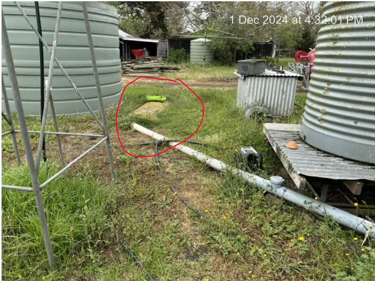
Existing Septic tank circled in red, showing above ground sewer inlet pipe from toilet.
