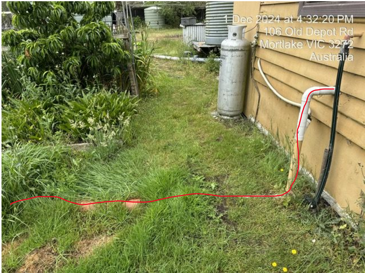
Grey water pipe discharging on top of ground to left of pic
