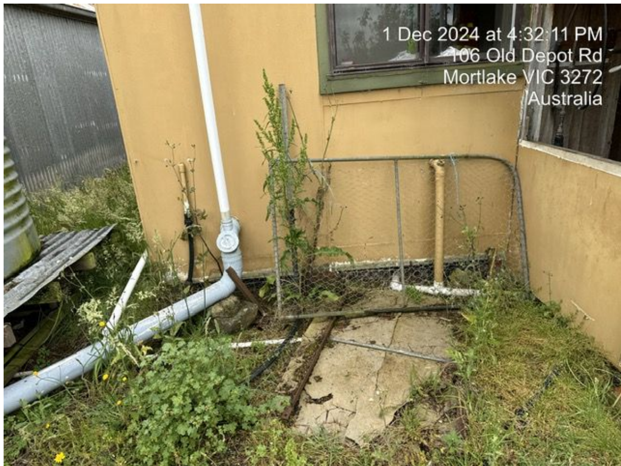
Toilet pipe on left and other waste pipes on the right. location
