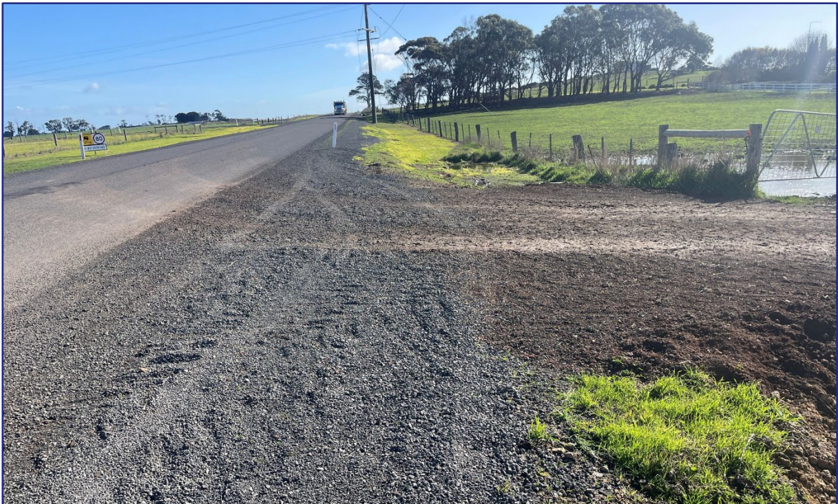
Figure 7: Photograph of Proposed Quarry Access
