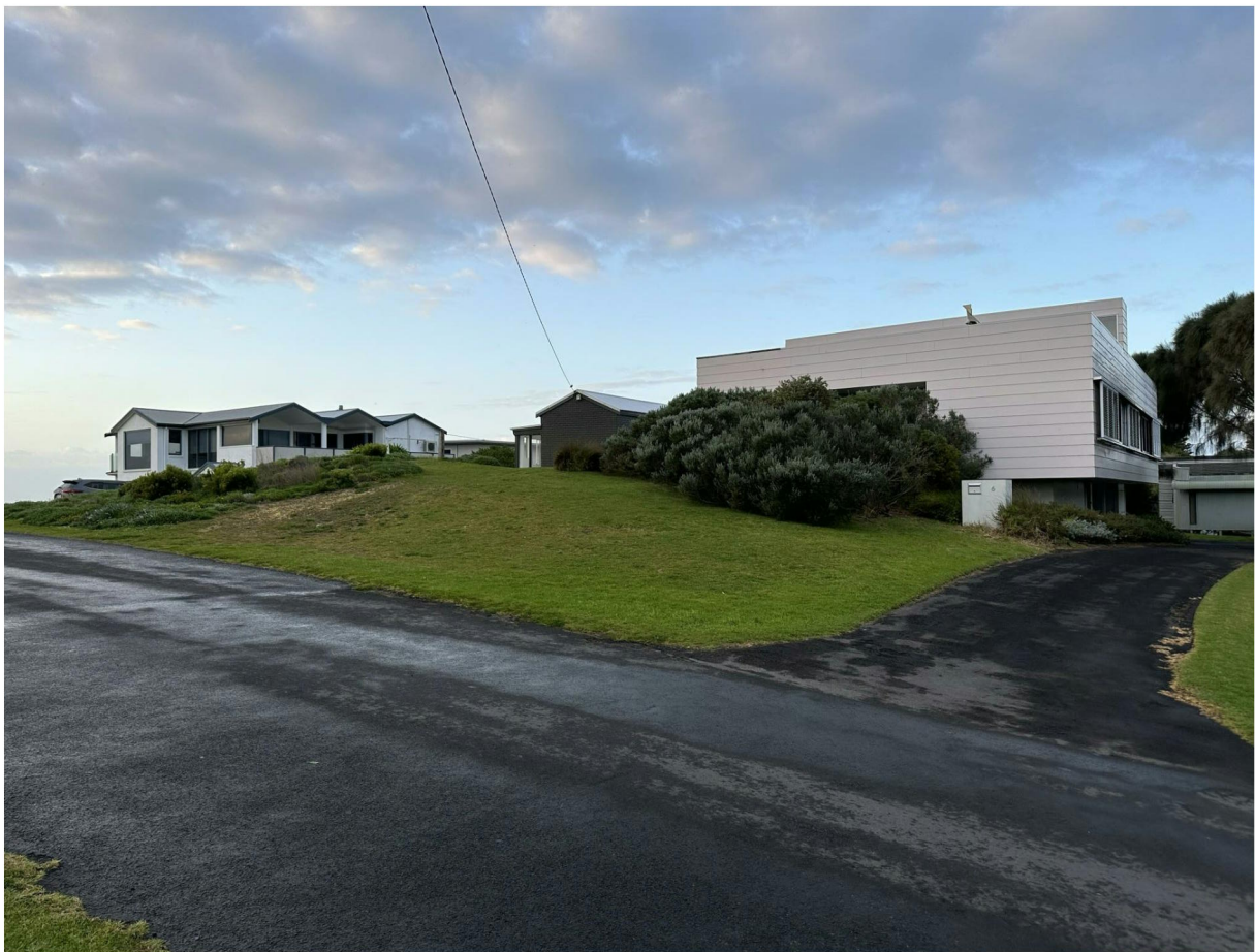
SUBJECT SITE: LOOKING SOUTH-EAST FROM NO.6 RITCHIE STREET TOWARDS NO.4 RITCHIE STREET
