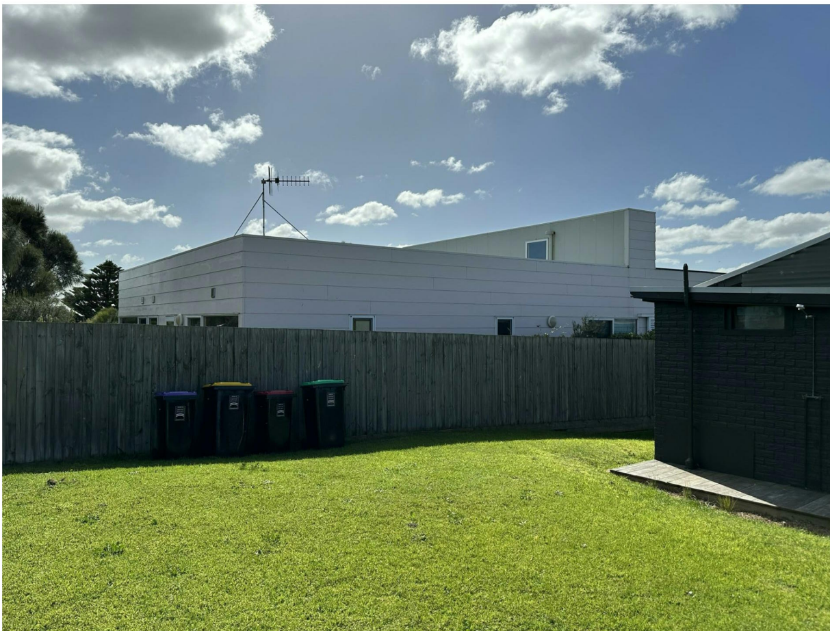
SUBJECT SITE: NO 6. RITCHIE STREET LOOKING SOUTH-WEST FROM NO.4 RITCHIE STREET
