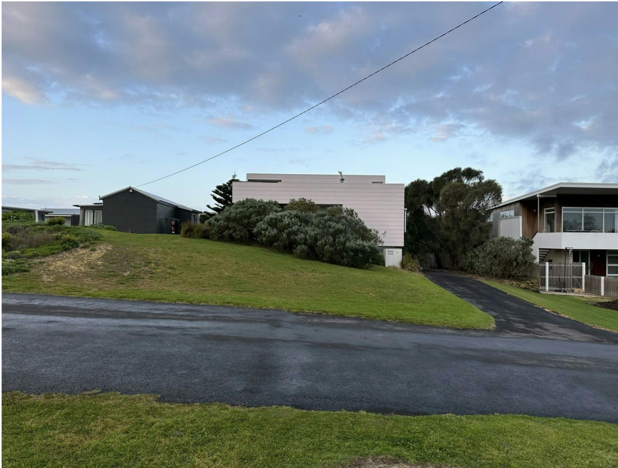
NO. 6 RITCHIE STREET - ADJACENT TO SUBJECT SITE
