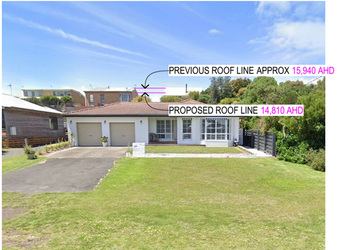
VIEW OF PREVIOUS DWELLING FROM 168C GRIFFITH STREET
