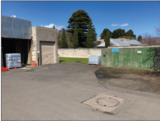
Figure 9 Rear 30/30A Sackville Street from laneway
