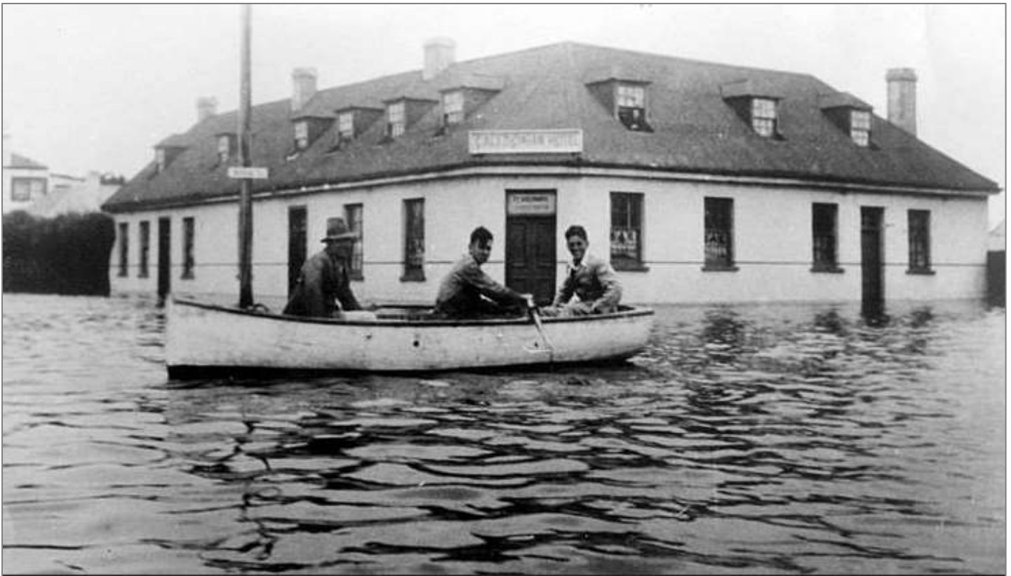
Figure 9. Flooding of the Caledonian Inn in Bank Street, Port Fairy in 1946, the largest flood on record.
