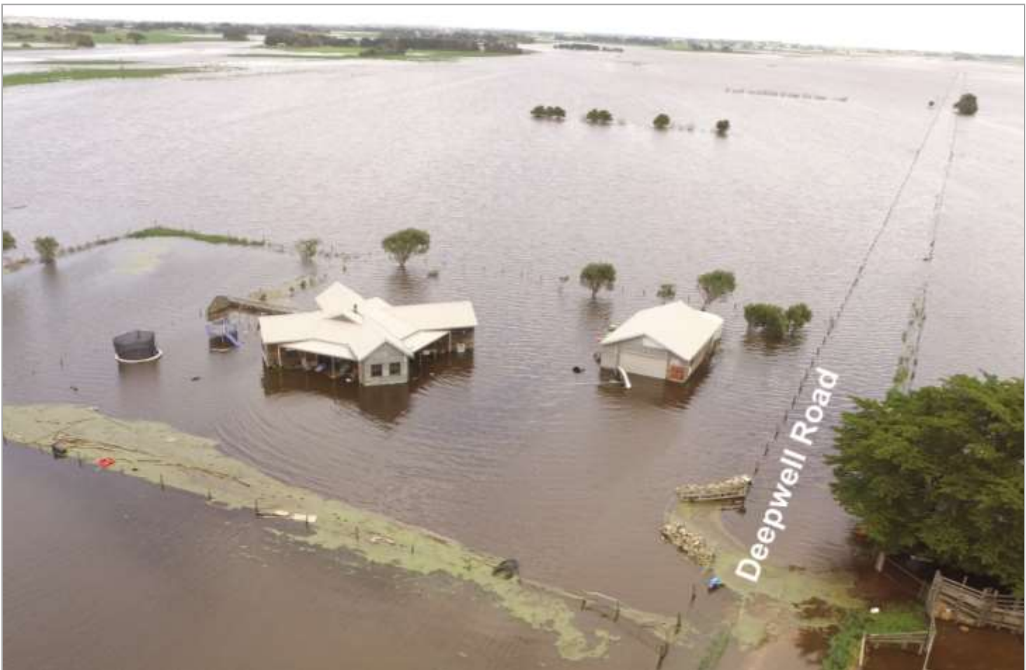
Figure 12. Flooding impacted a house in Deepwell Road, Crossley during the October 2020 event.
