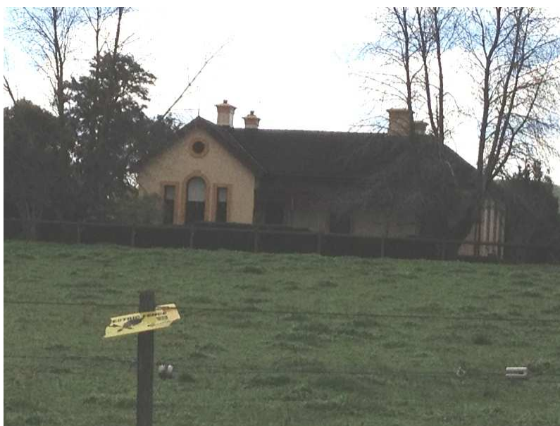
Presbyterian Manse Mill Street Mortlake
