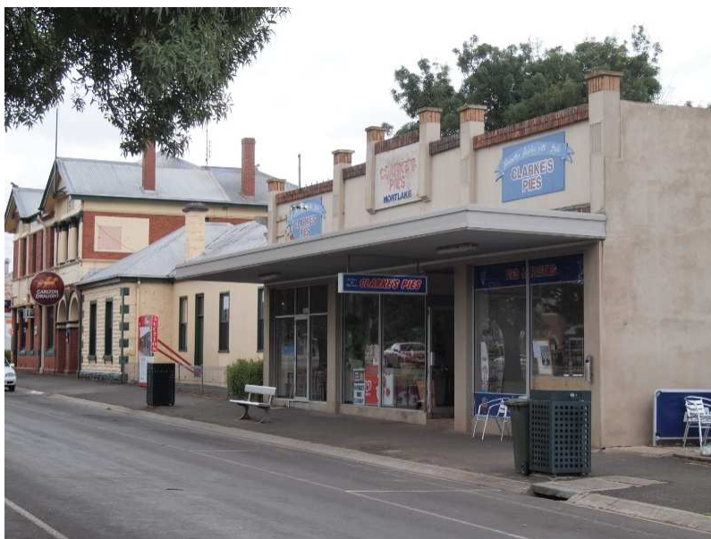
View looking west in Dunlop Street (north side of the street)
