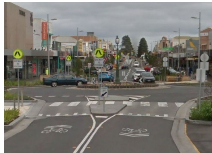
Examples of sharrow treatments that could be utilised on roundabouts within the town centre
