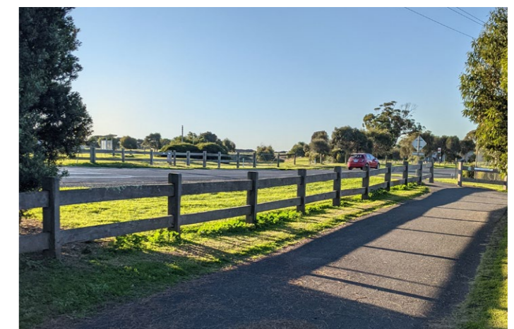
The Port Fairy to Warrnambool Rail Trail is a major recreational asset. Users are required to cross Princes Highway at grade which is a safety concern.
