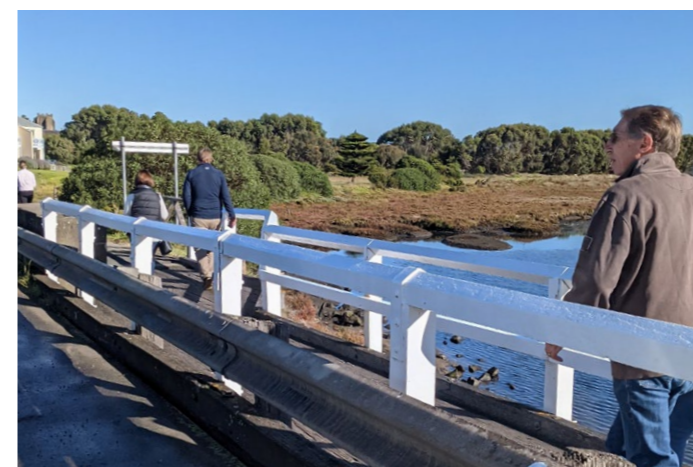
The footpath along the Gipps Street bridge is very narrow and not suitable for cyclists
