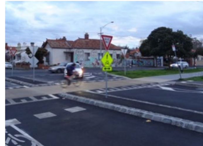
Examples of raised platform crossings that could be provided along Ocean Drive and other locations.
