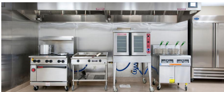
Figure 10 – Appliances on castors aids regular cleaning and sanitising processes.
