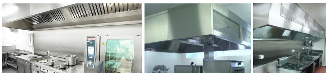
Figures 29-31 – Exhaust hoods shall be provided with approved metal washable dry type grease filters.
