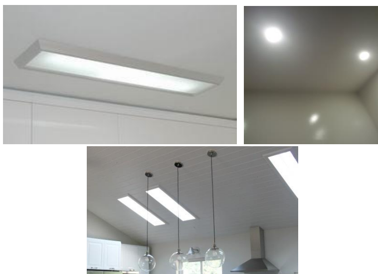
Figures 22-24 – For ease of cleaning, light fixtures should be recessed into the ceiling or fitted flush to the ceiling.
