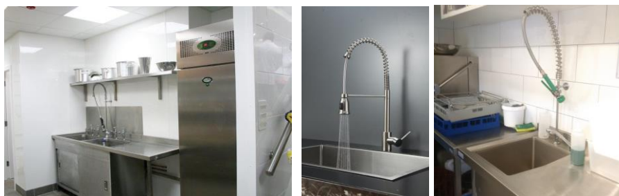
Figures 16-18 – Separate areas for washing food and washing equipment is required.
