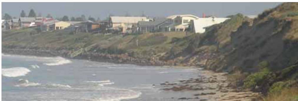
Figure 2-6 Rock Seawall Extended Past Connolly Street (2006)
