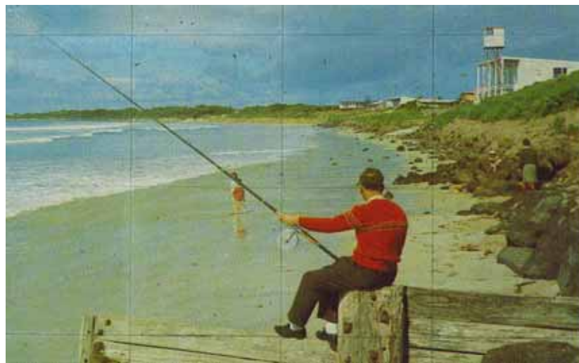
Figure 2-5 Commencement of Rock Seawall Construction at Surf Club (1965)
