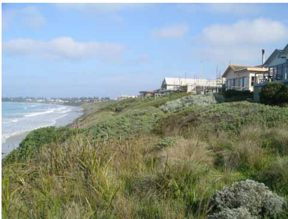
Photo 1: Development located on dune in erosion prone area
