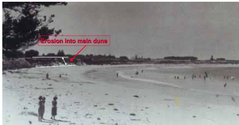
Figure 2-4 Erosion into East Beach Main Dune Approx 1930
