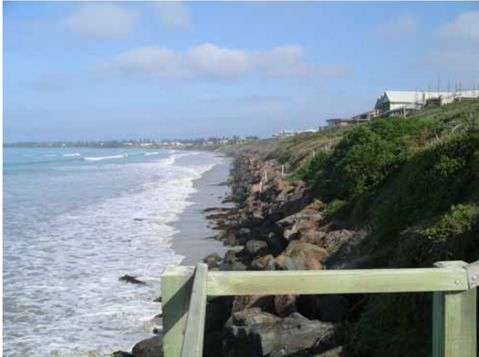
Photo 5: Seawall at East Beach has caused loss of usable beach
