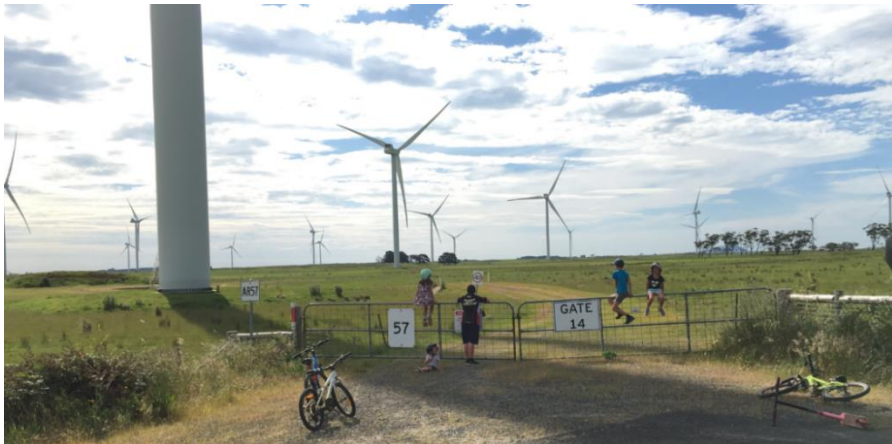
AGL – Gate 14 Gerrigerrup Rd. Macarthur Wind Farm. Unsecured wind power plant site – exposing the public to great risk.
