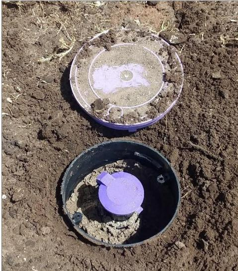
Figure 8 – Flush-valve installed at the end of each trench.
