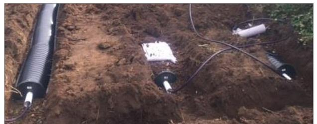
Figure 7 – Example of trenches and install of dosing pipe within 90mm slotted PVC and ReIn drain.
