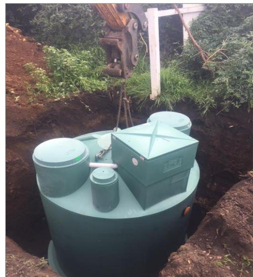
Figure 2 – Installing an OzziKleen RP10.
