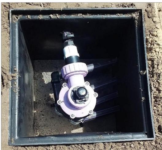
Figure 4 – The Rotavalve replaces distribution boxes.
