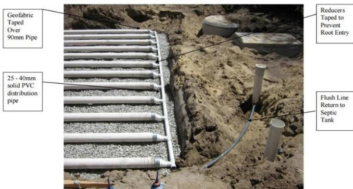
Figure 1 – Typical ETA configuration.
