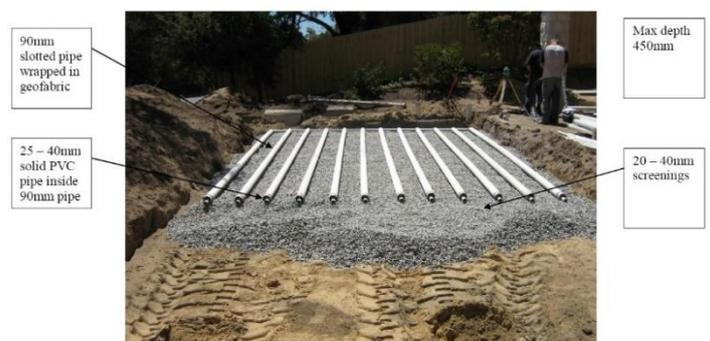
Figure 2 – Cross-section view of ETA bed.
