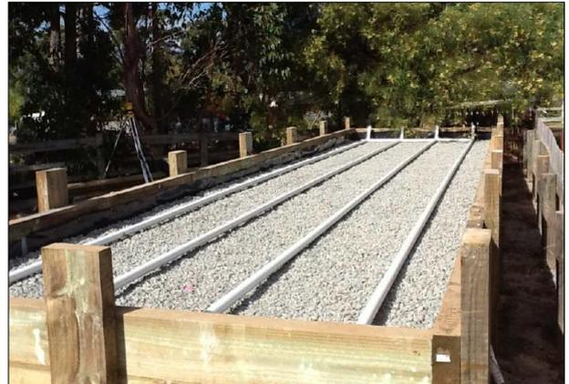
Figure 4 – Raised-bed ETA system. (Source: University of Illinois 2016)
