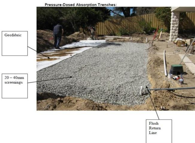
Figure 3 – Pipe-work covered with aggregate and geotextile fabric. (Source: Mornington Peninsula Council 2016)
