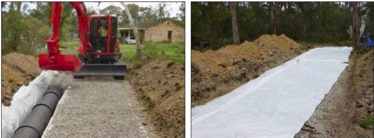
Figure 6 – Back-filling with aggregate.
