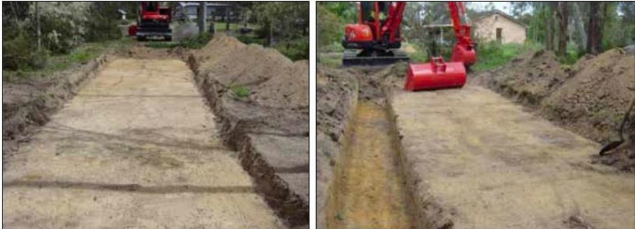
Figure 4 – WT & B initial excavation stage.
