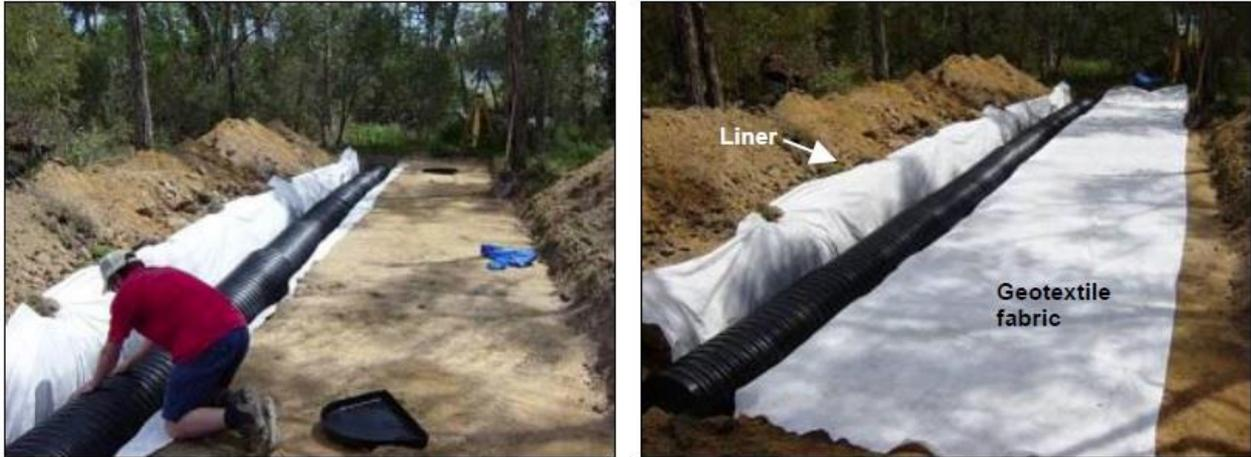
Figure 5 – Laying the geotextile fabric and arch drain.
