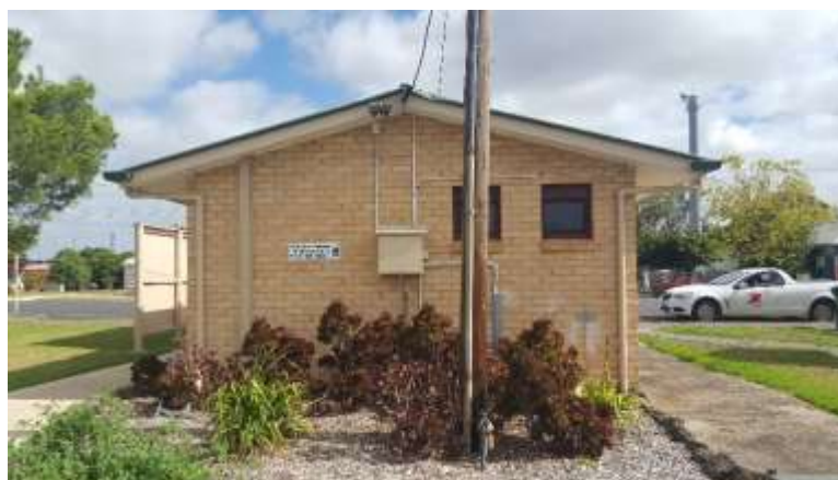
Current public toilet
