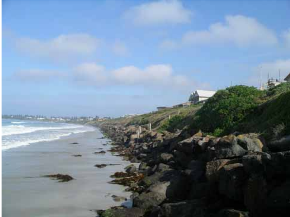
Photo 3: Seawall constructed in 1960s to protect development located on dune
