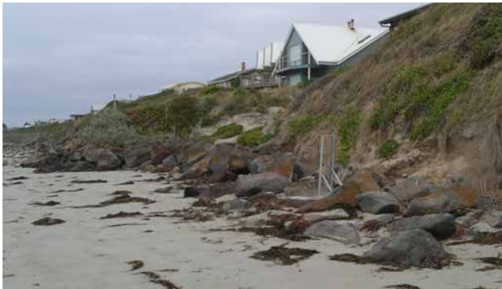
Figure 4-2 Northern End of Seawall of Sub-Standard Construction
