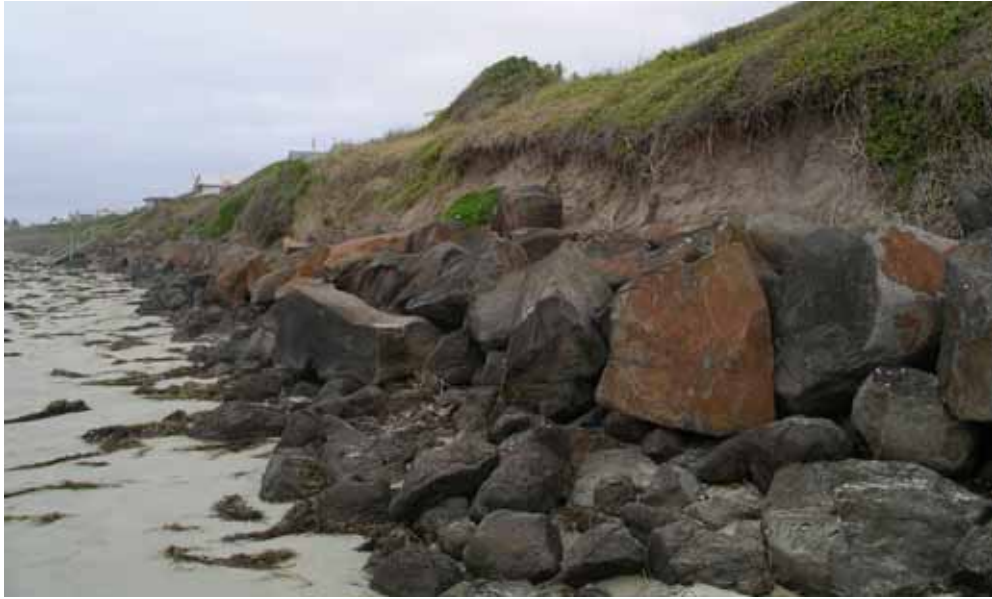
Figure 4-1 Section of Seawall of Sub-Standard Construction
