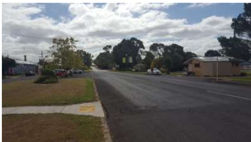
Existing High Street Road Reserve
