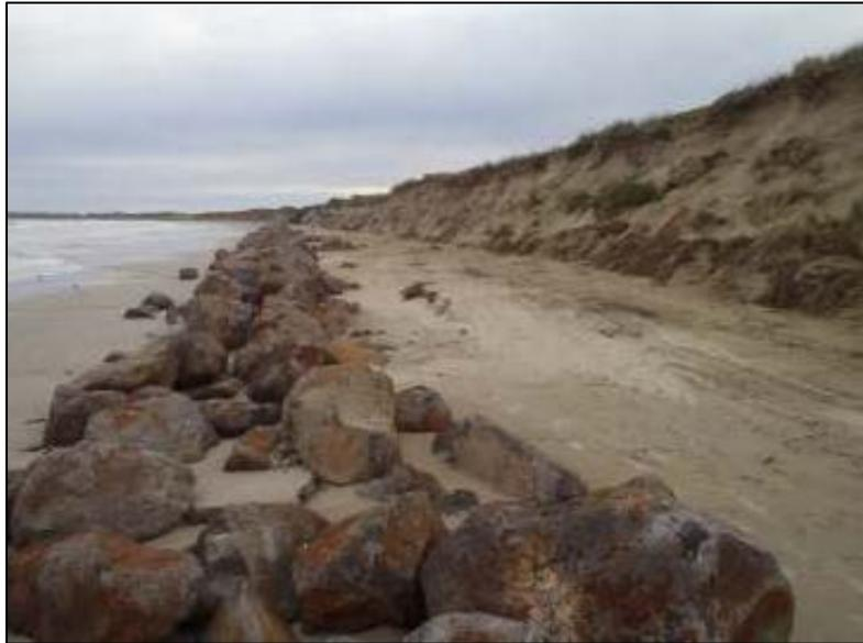
*Figure 13 Wave Energy Dissipation Structure (WEDS) at the Old Landfill East Beach*
